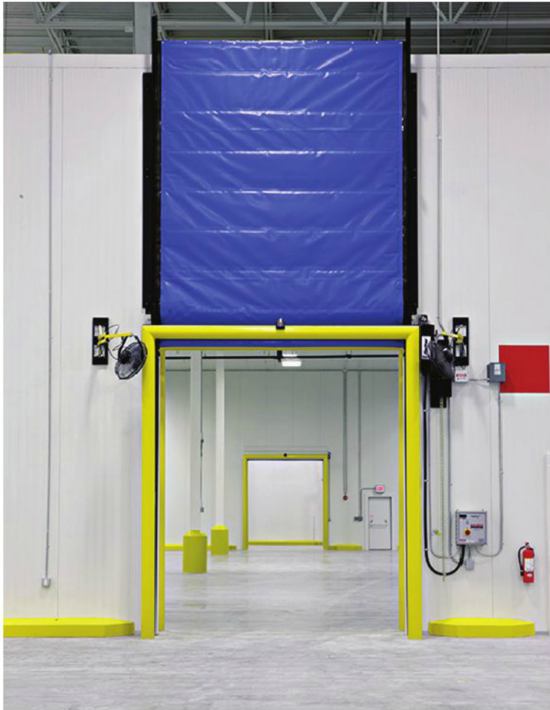
Some roll-up doors can operate as fast as 2.5 m per second—a rate which minimizes air infiltration and ensures optimal productivity.
